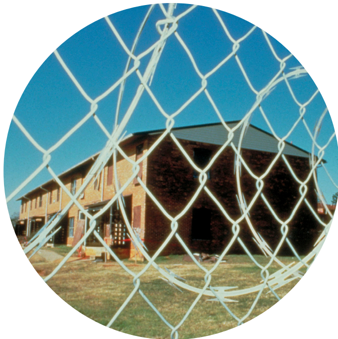
The former East Lake Meadows was defined by concentrated poverty, dilapidated housing, substandard education and rampant crime.
